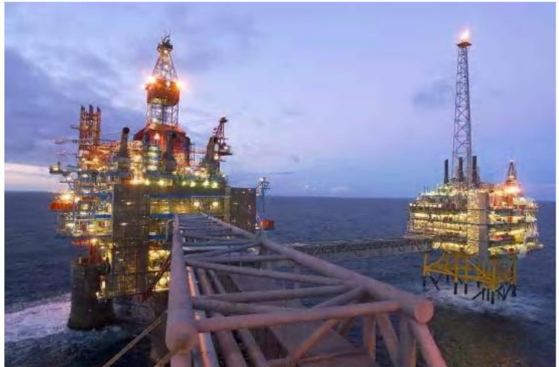
The Sleipner A integrated production, drilling and quarters platform is linked by a bridge to the Sleipner T gas treatment installation.
