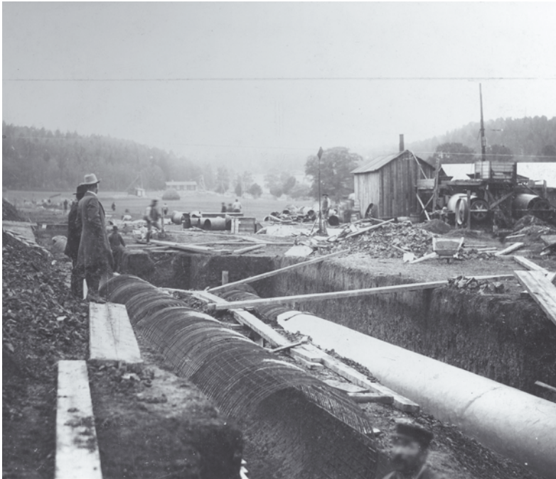
Norsborg plant under construction. Reinforced concrete was used for the first time for large structures in Sweden.
