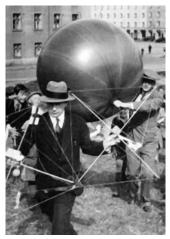
Finnish inventor Vilho Väisälä conducts experiments with his new radiosonde equipment, Tampere 1934.
